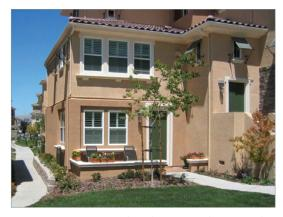
Figure 3.B.38: Units and porches can step down to grade to hide the parking podium behind
