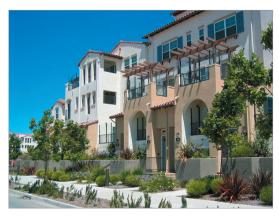
Figure 3.B.42: Use of Bays, Decks, and Trellises to Create Facade Variation and a Human-Scale
